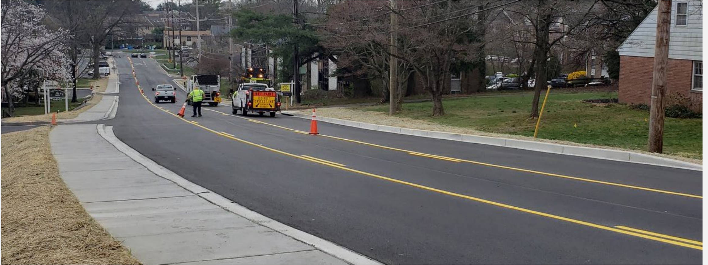
Sidewalk improvements and road reconstruction
